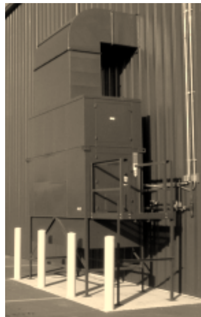
Installation with Optional Service Platform Shown
